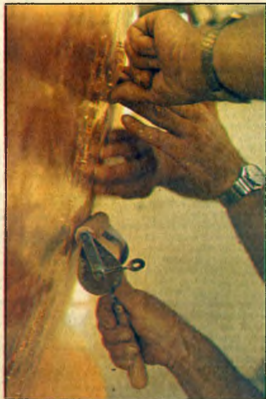
Clockwise from left, John Kozlovsky and Eugene Plishevsky finish the top of dome at St. Vladimir Memorial Church; small square of gold leaf is added and leaf is held and rolled into place by the two men.
