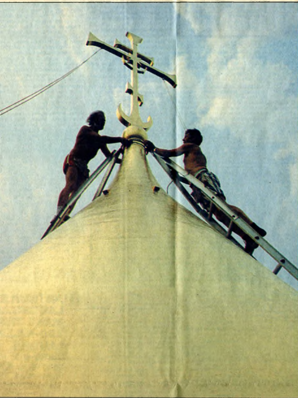
Clockwise from left, John Kozlovsky and Eugene Plishevsky finish the top of dome at St. Vladimir Memorial Church; small square of gold leaf is added and leaf is held and rolled into place by the two men.
