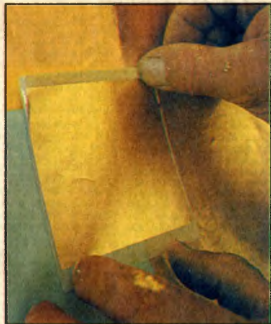
Clockwise from left, John Kozlovsky and Eugene Plishevsky finish the top of dome at St. Vladimir Memorial Church; small square of gold leaf is added and leaf is held and rolled into place by the two men.
